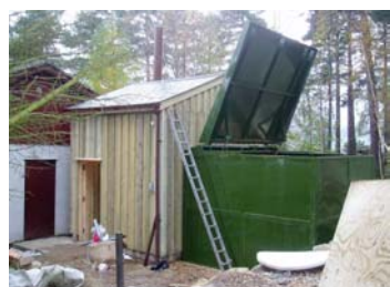
Fuel hopper under construction
