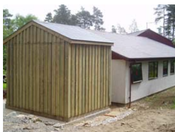
Fuel hopper under construction
