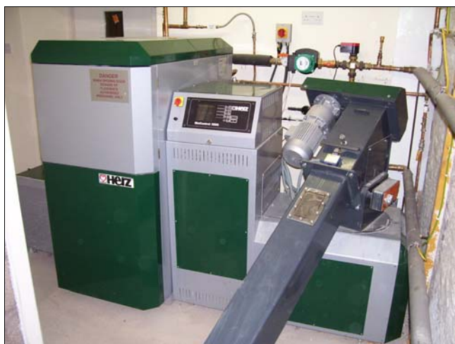
50kW Herz wood-fuel boiler from Austria installed by Wood-for-Warmth, Perthshire, Scotland
