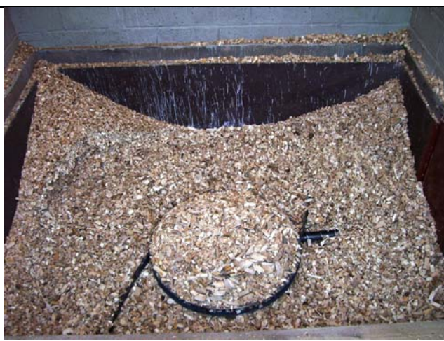
Wood-chip store below ground at the Wood-for-Warmth boiler installation in Perthshire, Scotland.
