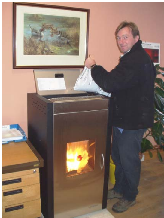
Figure 2 - loading pellets in a Calimax 10kW boiler
