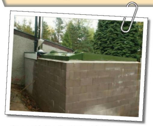
Fuel store and fuel handling: blockwork fuel hopper 3 x 3 x 2.25 (h) steel lid 3 x 3; hydraulic lift spring outfeeder to boiler feed screw
