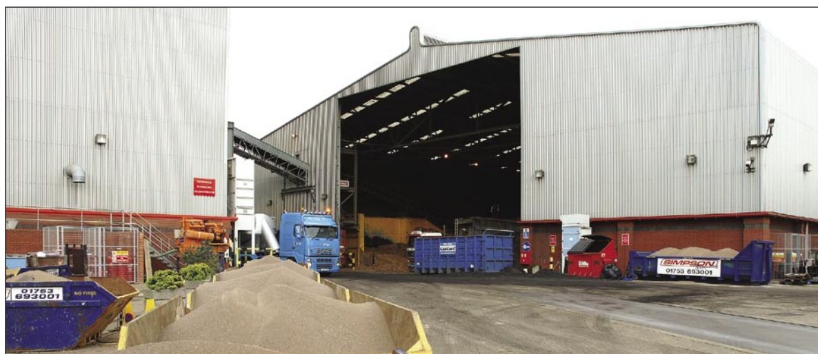
To the right, the front of the fuel store. The building on the left houses the biomass boilers. Between them can be seen the conveyor that connects the infeed system to the boilers.
